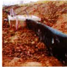
ReRoot 2000 has been installed prior to topsoiling in this infrastructure project
