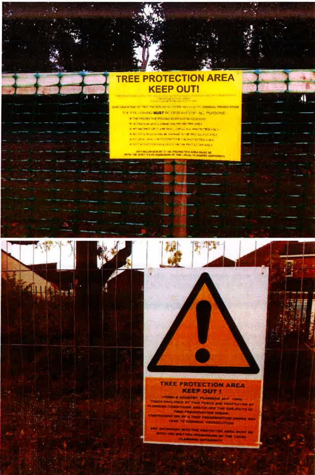
Figures 5 & 6: Examples of tree protection signage to be permanently attached to the root protection fence.
